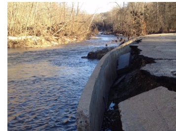
Damage at the Boat Ramp at Baptist Camp
